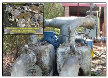
FIGURE 2: Vandalism, ageing infrastructure and insufficient maintenance of sewage infrastructure cause water pollution, which contributes to the eutrophic conditions in receiving water resources.
